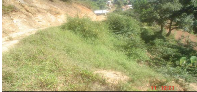
Village roadside stabilisation using forage species
