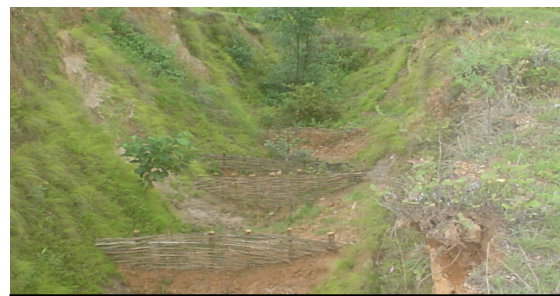
Gully control using vegetative measures
